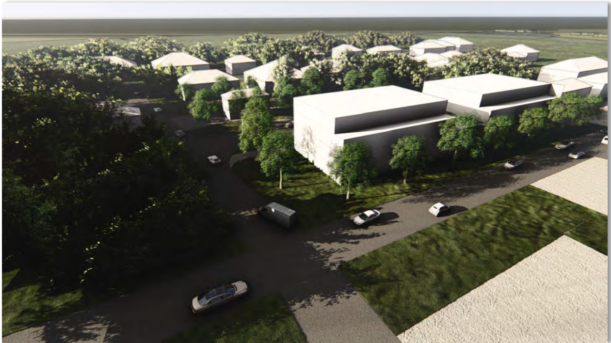
View Looking Southeast at Grey Road 19 and Craigmore Crescent Intersection
