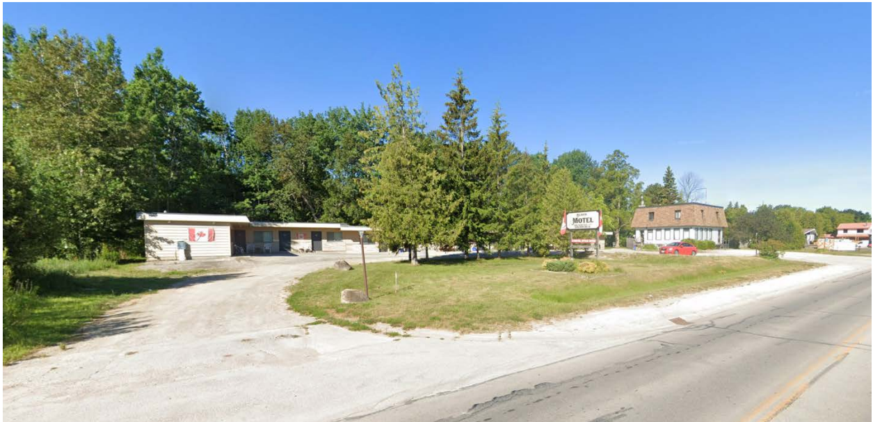
Potential Intensification Site C on the South Side of King St. E.
