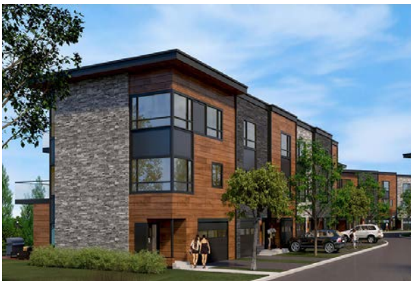
Towns of Thornbury (Under Construction)
